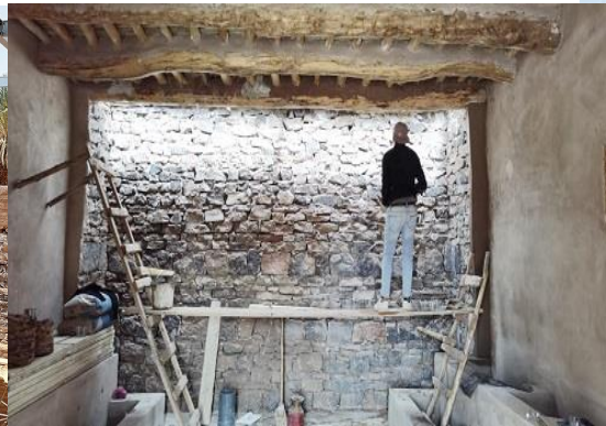
Finishing touch to Waterreservoir
