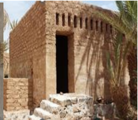
One side of eco-toilet complex
