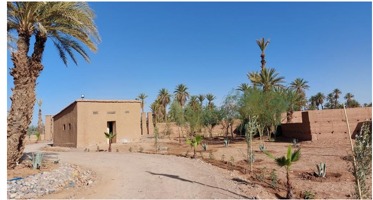
Classroom on top of Waterreservoir
