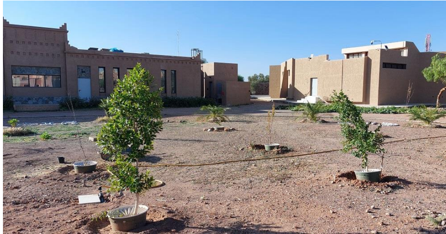
Hotel & Guide school ISTAHT in Ouarzazate
